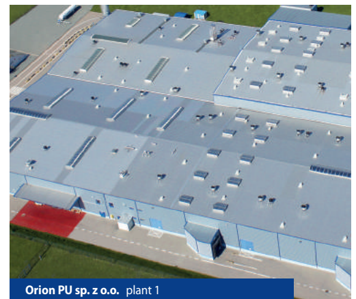
Orion PU sp. z o.o. plant 1
